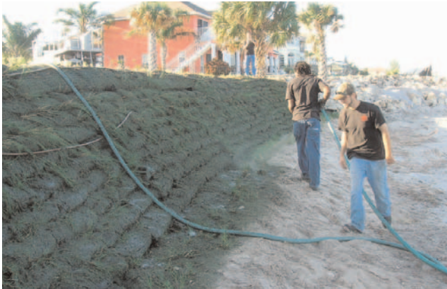
Hydroseeded shoreline wall
