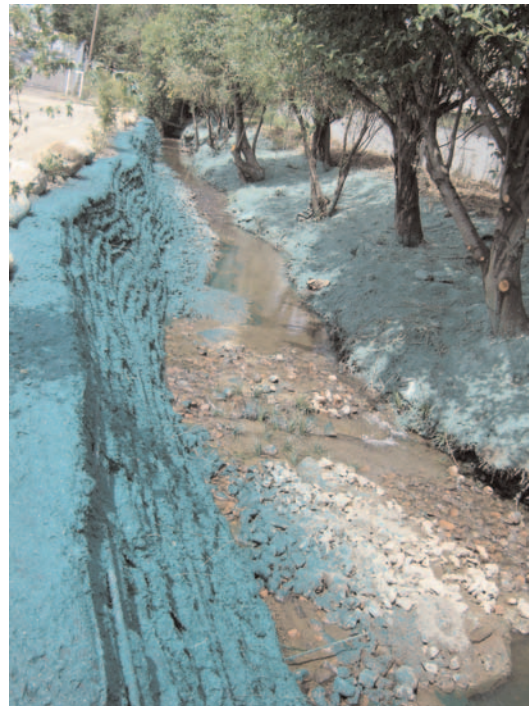
Hydroseeded streambank wall
