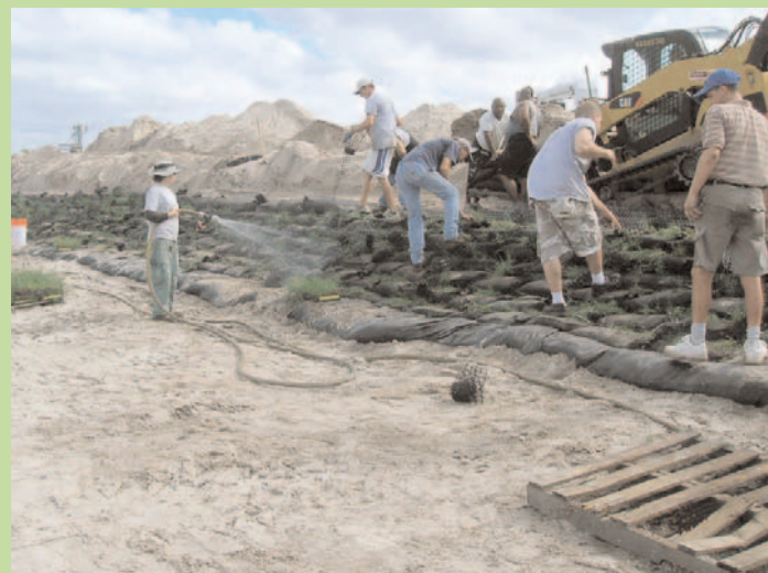
Installing the wall
