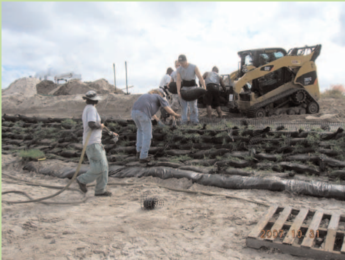
Installing the wall
