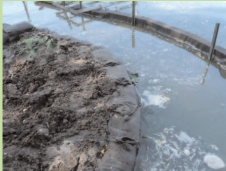
Building the wall
