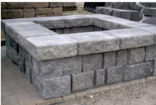
Finished Fire Pit, Front View
